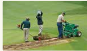
Core Collection and Removal
